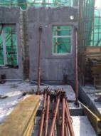
The facade and bay window units have precast concrete to provide the structure behind the GRC skin which in turn provides the desired architectural finish.
