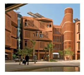
The GRC façade has been designed as a series of curved balconies in a wave pattern that alternates on each floor so when the balcony on one floor is convex the balcony immediately above is concave.
