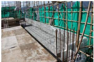
The balconies are aligned together with the internal formwork used for the floor slabs to enable a homogenous floor slab to be poured.
