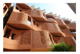
These balcony units are highly complex with the GRC units including openings for lighting; GRC permanent form panels to receive the screed for the in-situ balcony floor above; built-in GRC slatted soffits and ceilings (to look like timber slats, which were originally to be manufactured from renewable source timber); curved GRC panels; and curved GRC screens, all to millimeter accuracy.
