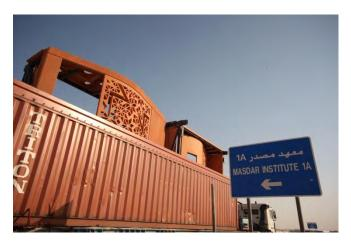
Erection of these balcony units originally would have taken up to 10 days for each Residential unit but subsequently the GRC facade modules were fixed in place in only 2 hours.
